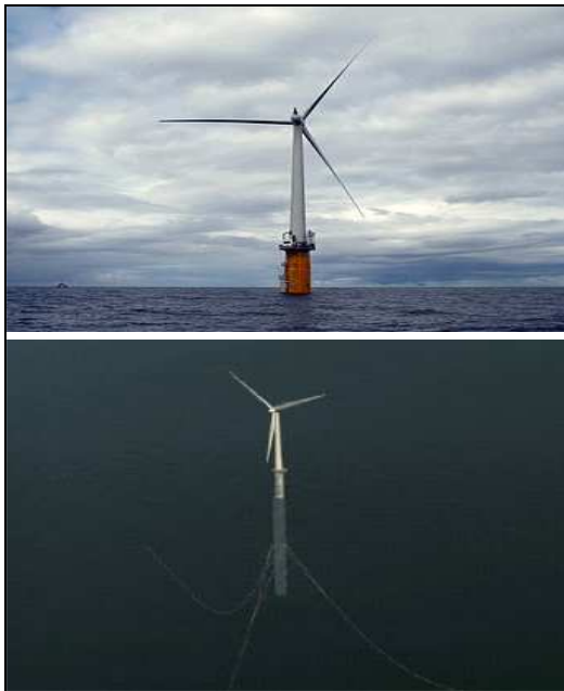
Figure 5: Example of an offshore wind energy device; the Hywind device, developed by Statoil (Photo: Trude Refsahl / Statoil; Illustration: Still shot from animation: Hywind assembly) www.statoil.com
