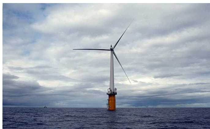
Figure G: Photograph of Hywind floating wind turbine under testing (designed for use in water depths of 120–700m), an example of the type of innovative technology which will need to be developed to facilitate exploitation of the extensive combined resource in deep waters. (Photo: Trude Refsahl / Statoil)
